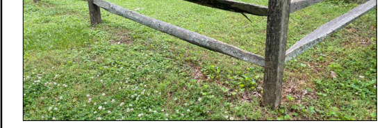
Split Rail Fence to delineate perimeter/boundary Precedent image of on-site cedar two-rail split rail fence
